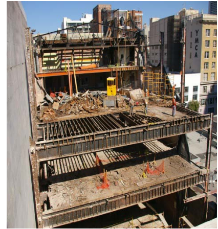
^ Demolition In Progress (from back)
