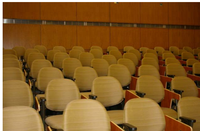
Moot Court Renovation - In Progress
