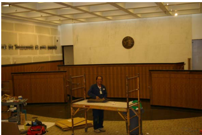
Moot Court Room Renovation - In Progress
